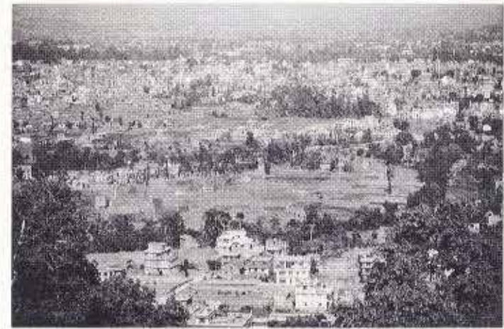
The inflow of migrants and the booming tourism, carpet and foreign aid sectors have led to a sprawl of Kathmandu. The traditional "compact city" is breaking up while distances between homes and jobs are increasing. In the absence of effective land use control Kathmandu is spreading over fertile paddy fields.
