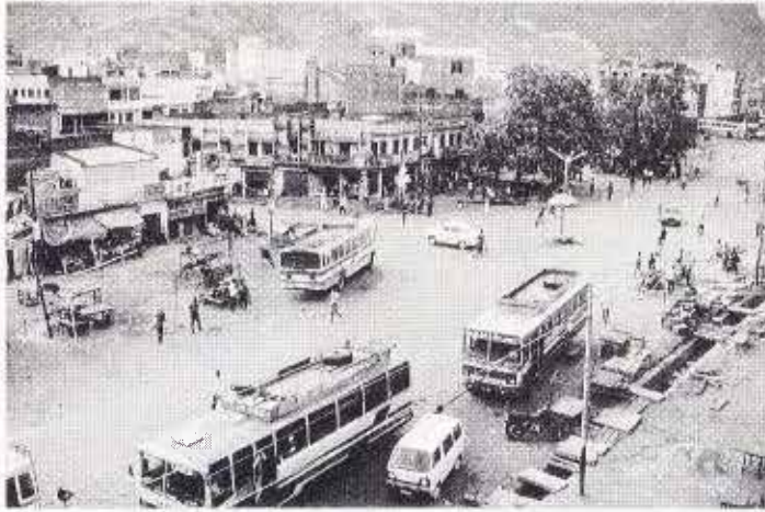
Butwal: the fast growing city is located at the junction of the east-west highway and the highway connecting Pokhara with the Nepali/Indian plain. The metal workshops in Butwal, originally initiated by foreign aid (UNM), have grown to a significant business offering employment in increasingly specialized fields (e.g. overhaul of buses and trucks). Having faced saturation, Butwal's industry is now diversifying into spinning industries.
